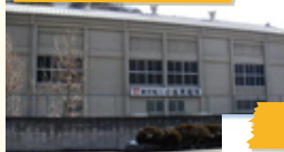
Komatsu Power Station
